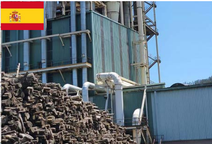
Spain wood processing plant Coepo APF-4L-400V, 3P4W,2600A Coepo SVG-4L-400V, 3P4W,200Kvar
