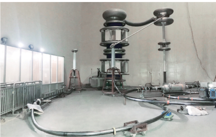
High voltage test
